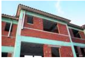
To external walls
