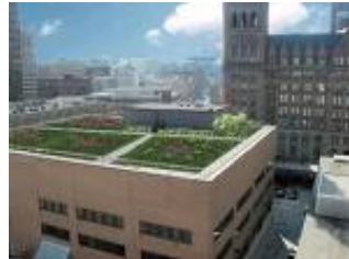
Vegetated Green Roof
