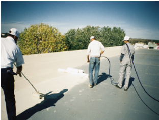
Cool Roof with white reflective coatings
