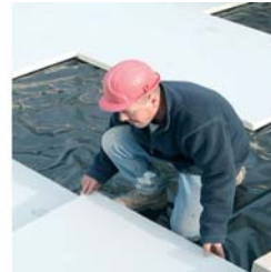
Thermally Insulated Roof
