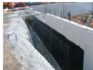
SA Applied to Retaining Walls and Covered with Protection Boards.
